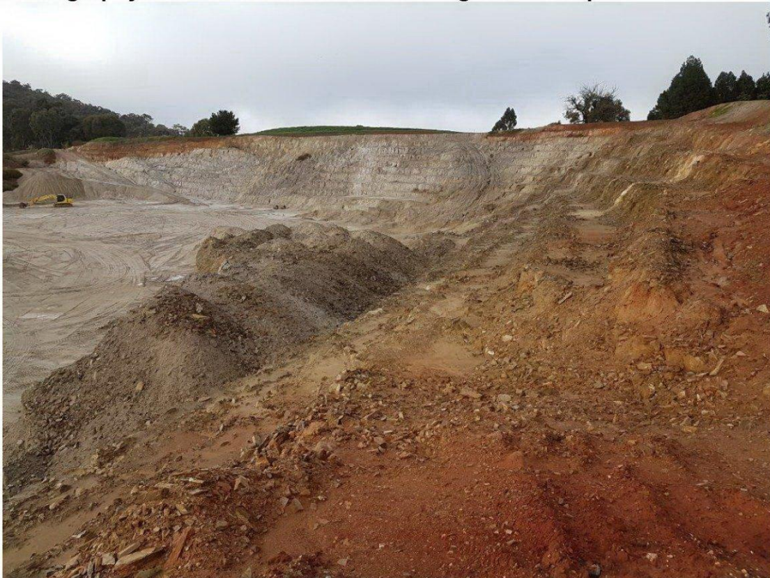
Photography 8: Stable batters and benching in current pit
